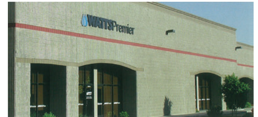
The acquisition of Premier Water Systems ushered Watts into the RO technology for purifying water.
