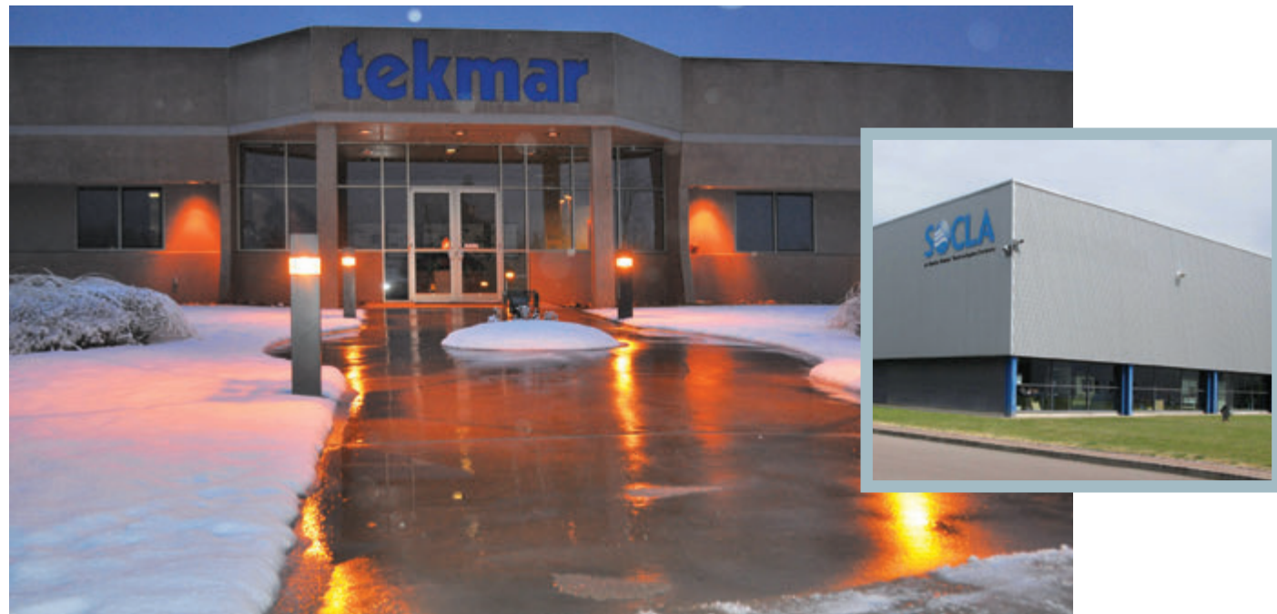
Left: tekmar Control Systems in Vernon, BC, Canada. Right: Socla’s main plant in Virey le Grand, France.
