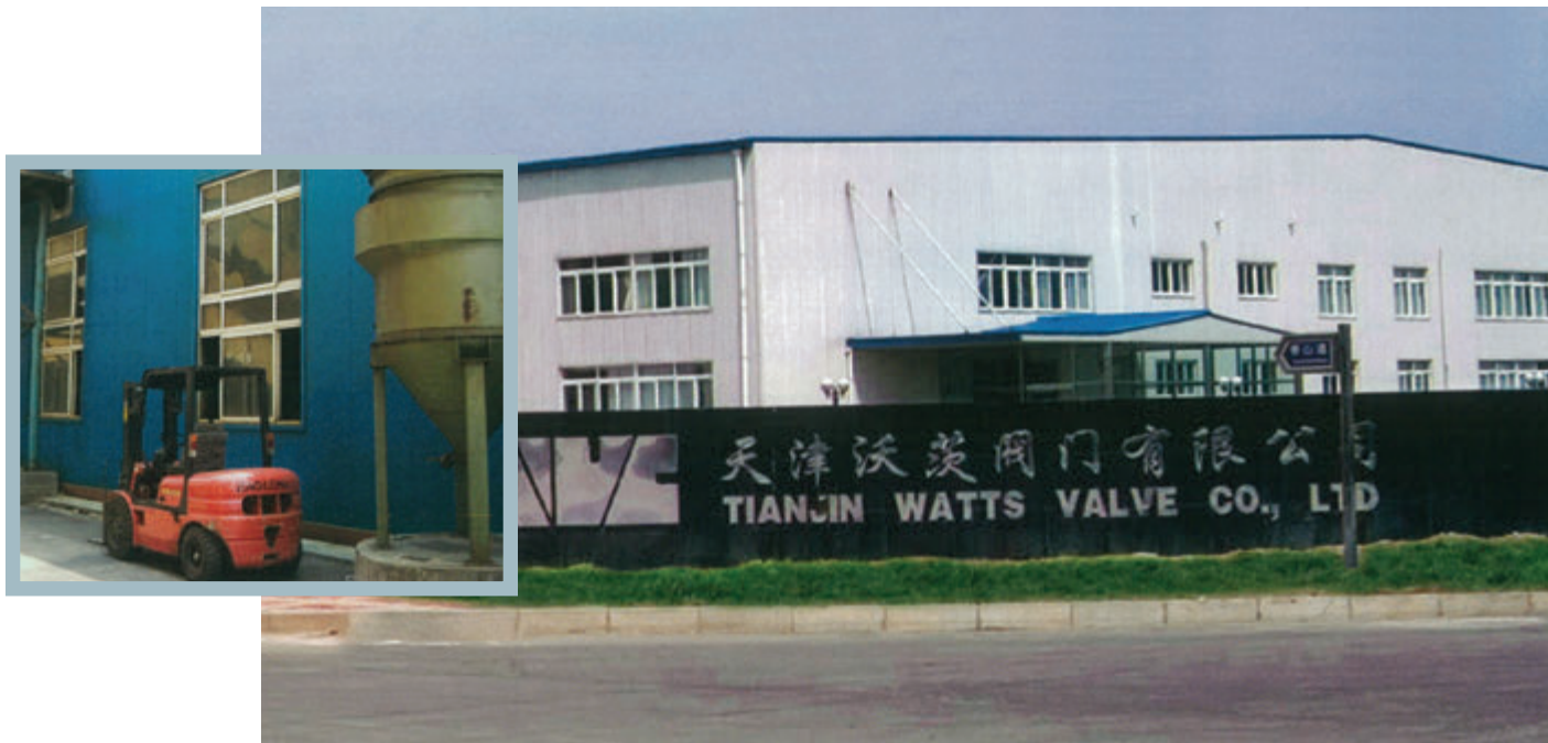
Watts opened its new state-of-the-art 125,000-square-foot Tianjin Watts Valve Company plant in the fall of 2003 to machine the castings from the Tianjin Watts Bronze Foundry. The Tianjin Watts Bronze Foundry, with a capacity to produce more than 200 tons of finished castings per month, was an outgrowth of Tim Horne's vision.
